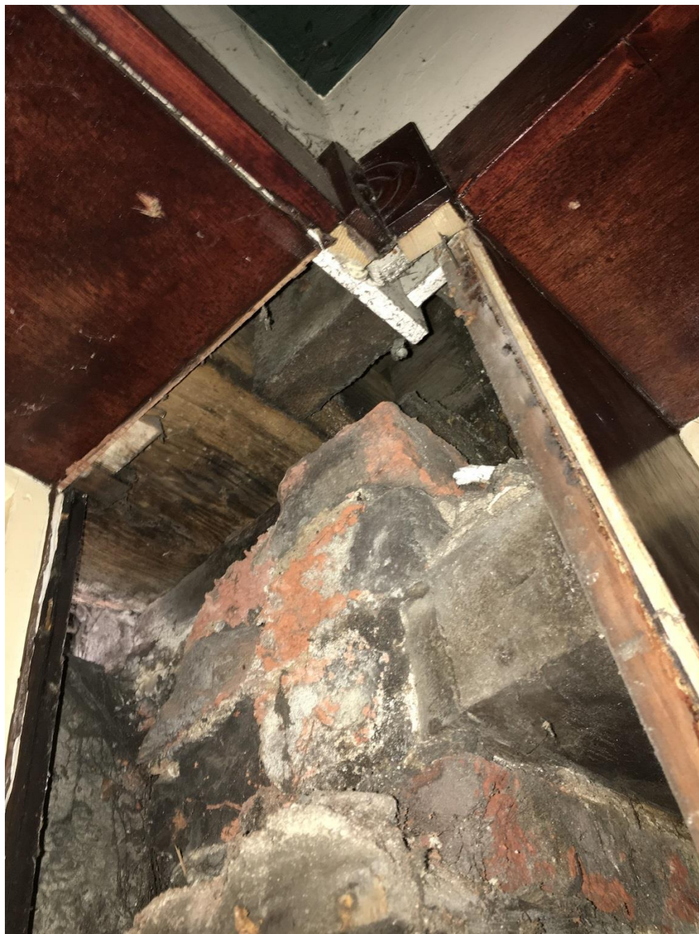
Image 6: Timber boarding at window head level
