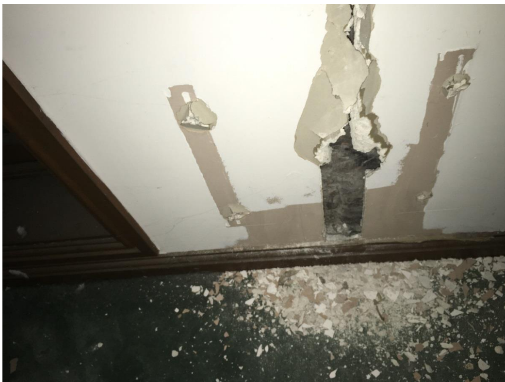
Image 1: Modern plasterboard and skirting.
