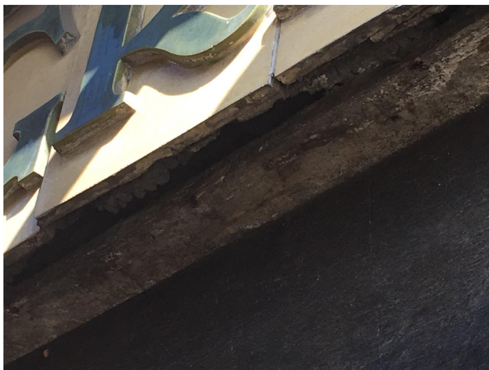
Image 8: Timber Boxing Construction behind signage tiling
