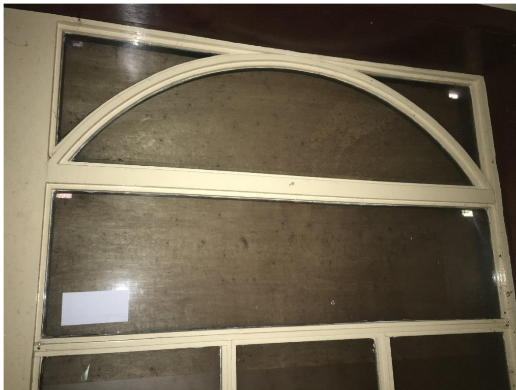
Image 4: Softwood fixed pane windows to ground floor.
