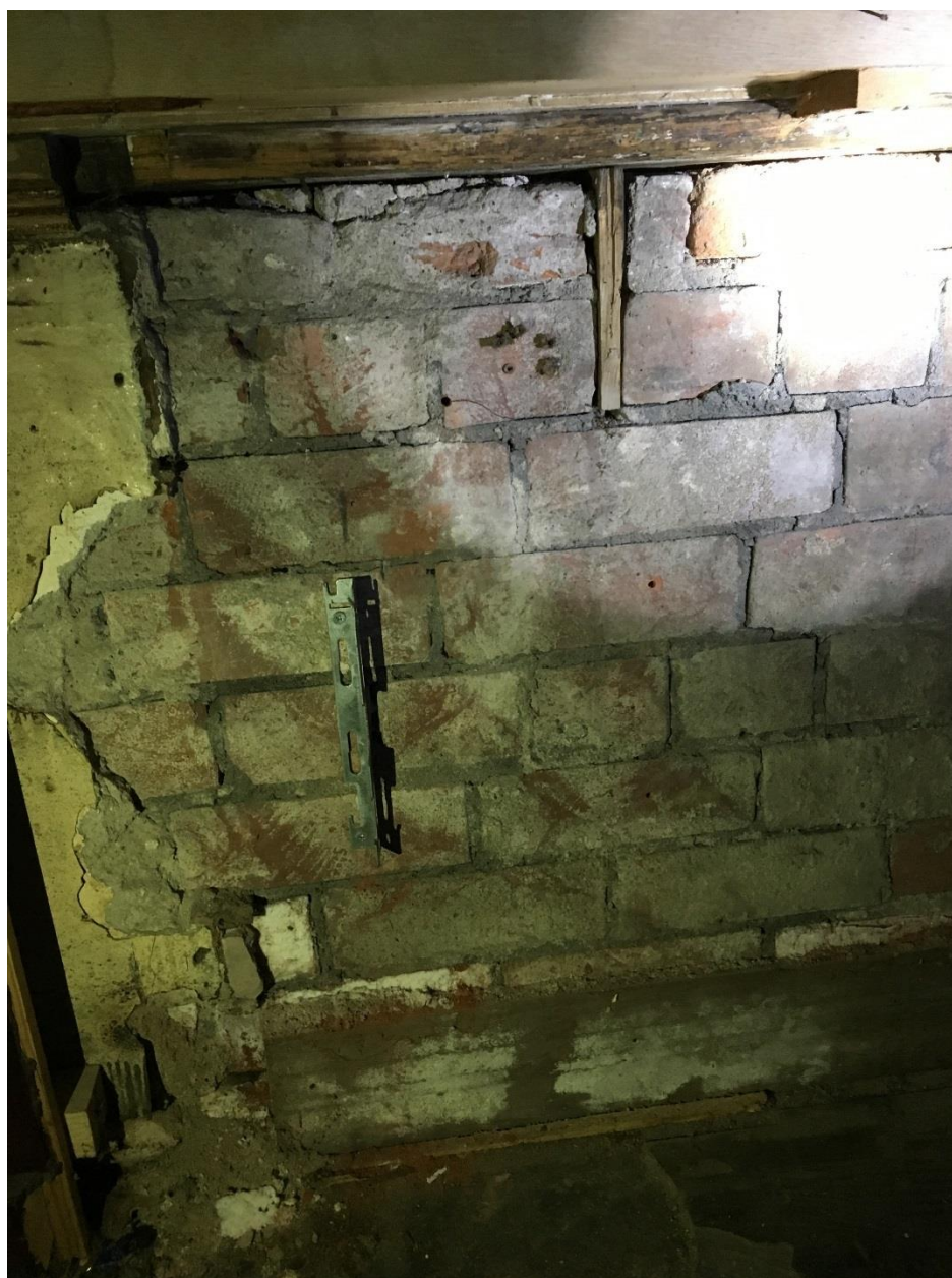
Image 2: Lower level brick at ground floor with visible headers.
