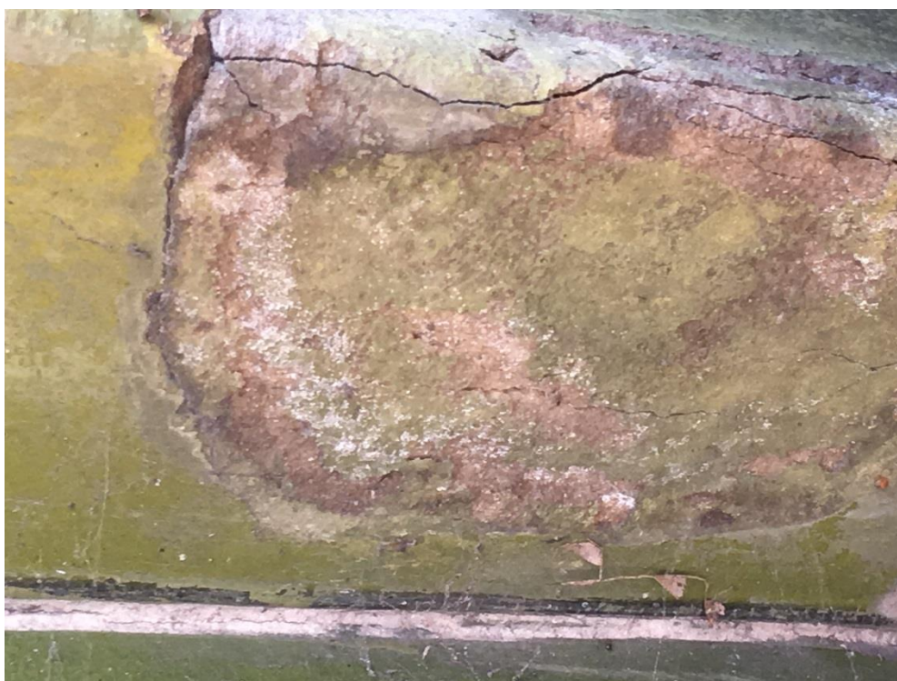
Image 12: Green coloured repair to glazing finish
